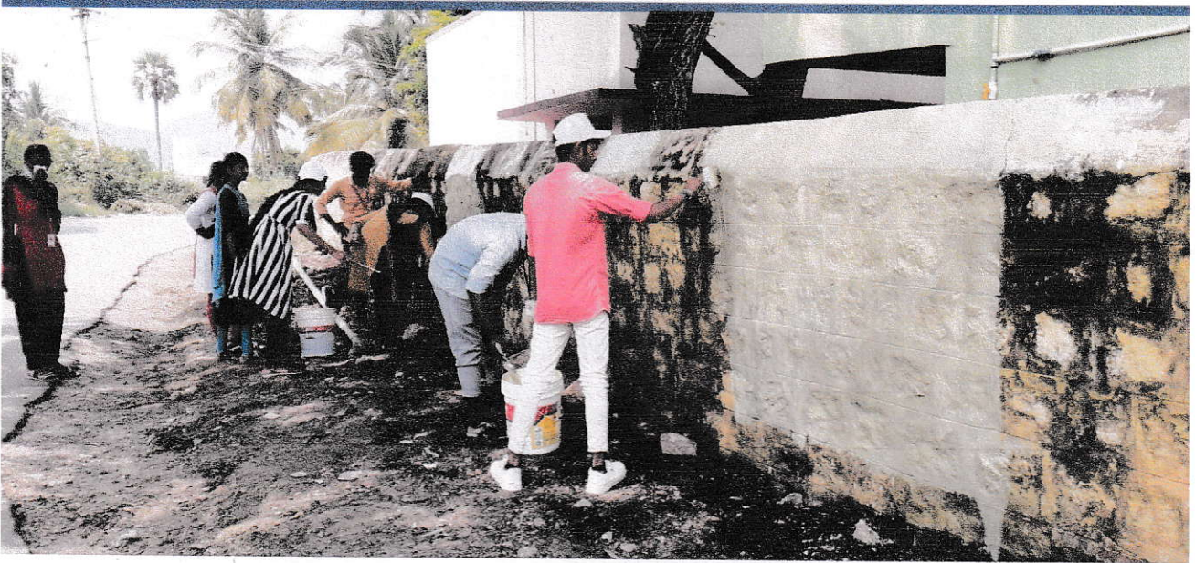
Students engaged in whitewashing activities in School, Devannagoundanur village
